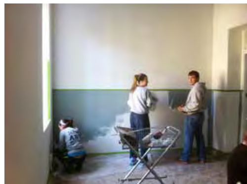
Prep work for this museum exhibit also involved painting. One challenge for mounting were two-foot thick masonry walls from before the Civil War.
